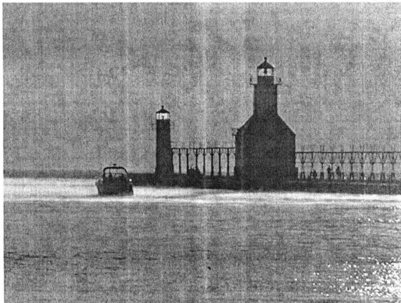
Figure 1. St. Joseph North Pier Lighthouse (Source: Emily B. Starke, 2001; www.michigan.gov )
